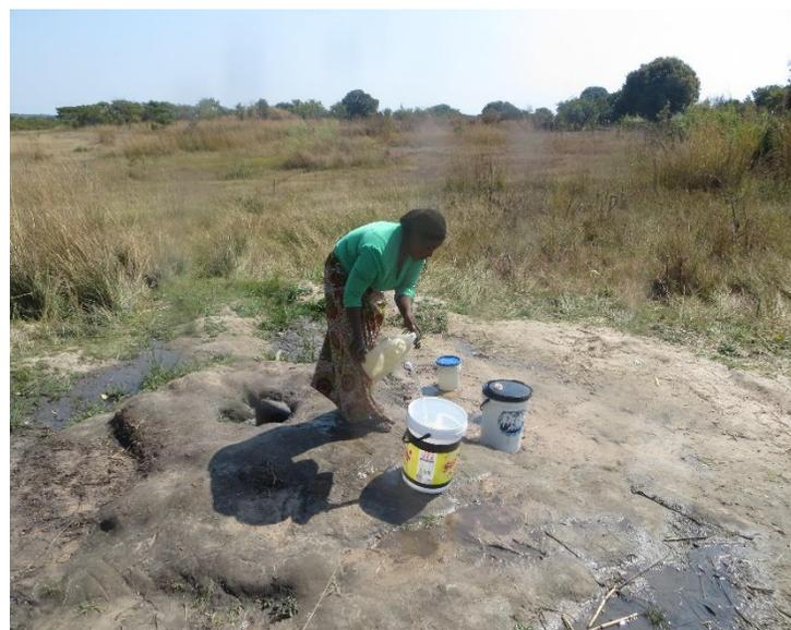
Further investigation showed that the borehole needed to be rota jetted to remove siltation and deepen it and the pipes, rods and handpump required replacement.
